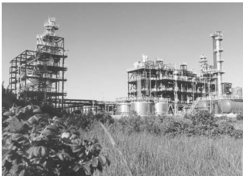
MDI manufacturing plant (figure by courtesy of Huntsman Polyurethanes)
